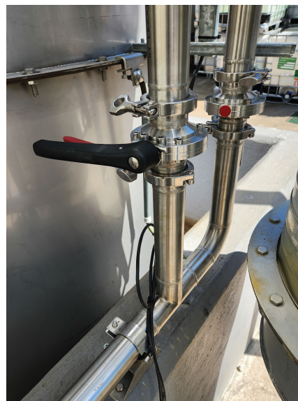
Stainless steel reticulation and process piping supporting contaminant treatment and reliable long-term scrubber operation during system use.
