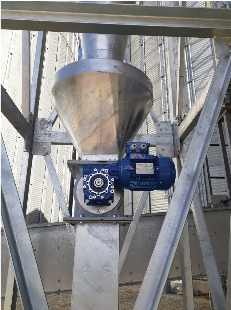
Rotary valve discharge system maintaining continuous material removal while preserving cyclone efficiency.
