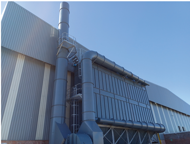
Screw conveyor system for controlled removal of collected particulate matter.
