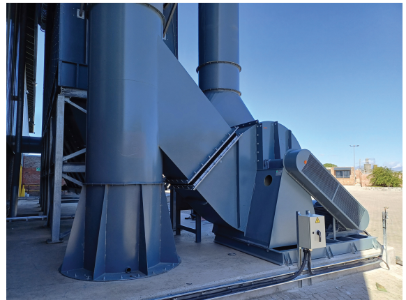
Baghouse filtration unit designed for acidic, high-humidity galvanizing fumes.
